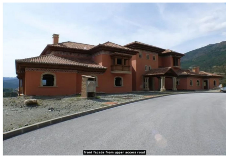
from facade from upper access road
